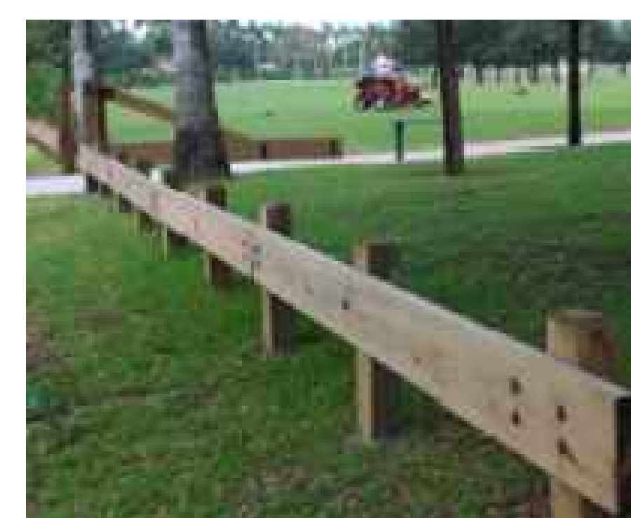
Wood Guard Rail Not to Scale
